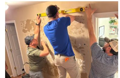
Hope Mountain Church volunteers helped repair sheetrock and repaint areas on our bottom floor to continue updating our office.
